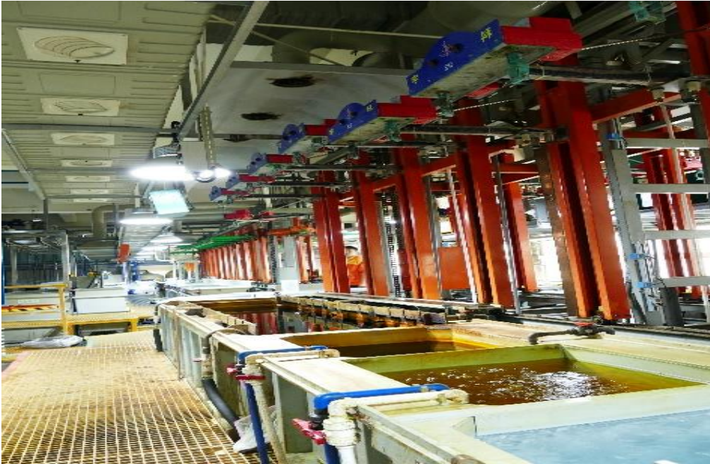
Fig.1 Example of exhaust gas emissions in Longxi Electroplating Park
